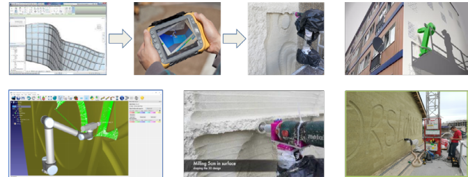
Collaborative robot for façade retrofitting by on-site 3D rendering and milling
