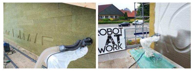
Milling with the robot (left); Spraying on the finishing layer
