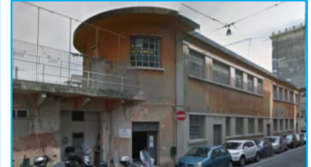
Deep renovation of historical nursery building in Genova, IT
