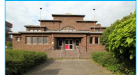
Transformation of public spa building to dwellings in Hürth, DE
