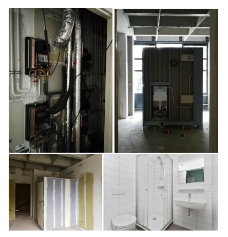
Prefabricated **bathroom units**
