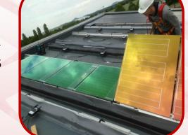
Covered solar heat collectors using colored NIR transparent glass
