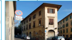
Deep renovation of historic residential building in Florence, IT
