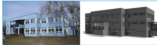
Deep renovation of public nursery building in Warsaw, PL
