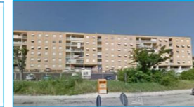
Deep renovation of residential building in Ancona, IT
