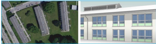
Residential district renovation in Odense, DK
