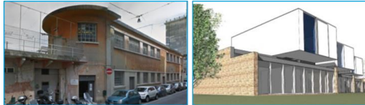
Deep renovation of historical nursery building in Genova, IT
