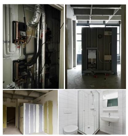
Prefabricated bathroom units
