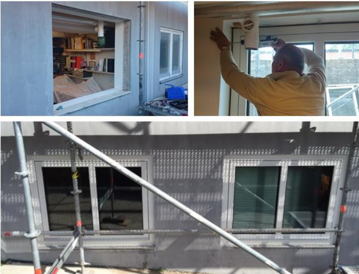
Figure 26: Installation of first Smart Window prototype on building in Sweden
