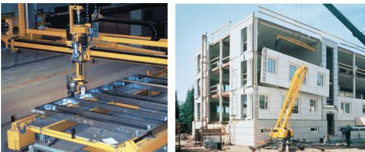
Figure 9: Prefabrication of steel frames and installation 8
