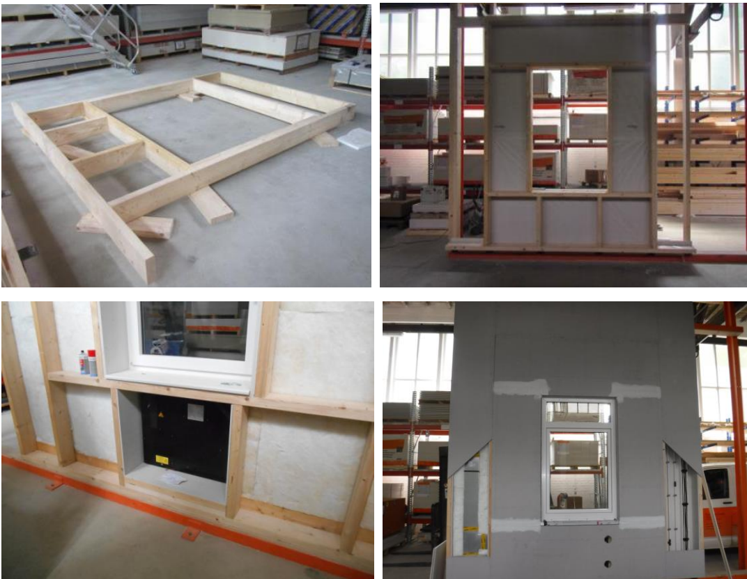
Figure 15: Prototype of multifunctional façade panel constructed by Fermacell
