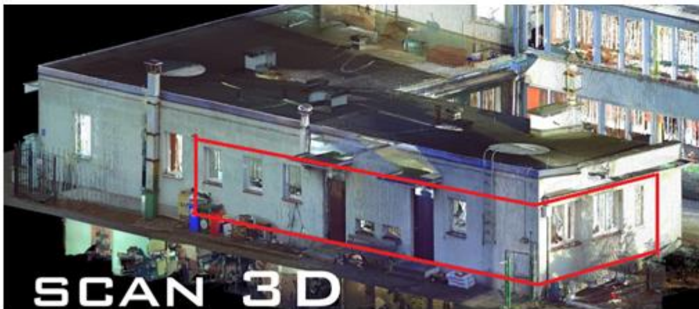
Figure 29: Gdynia demo building – proposed windows for replacement
