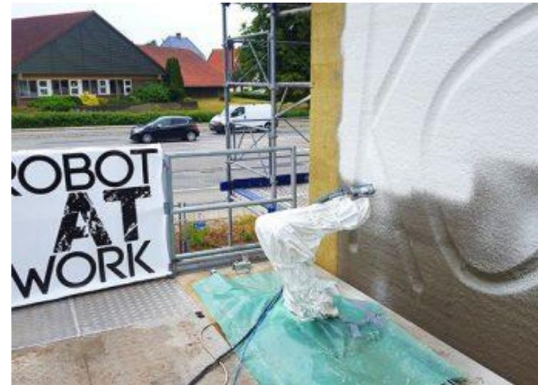
Milling with the robot (left); Spraying on the finishing layer
