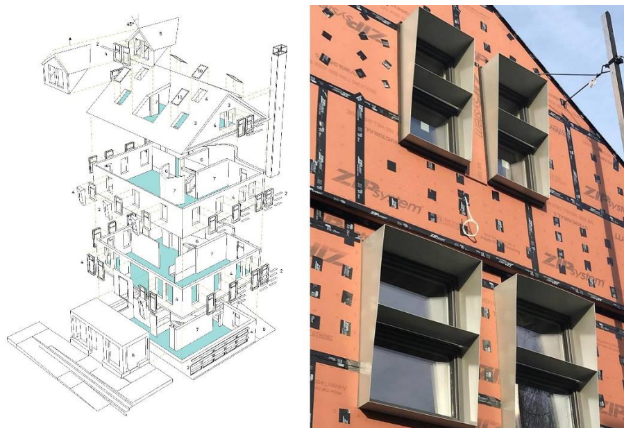
FIGURE 2. LEFT: BUILDING INFORMATION MODEL BREAKDOWN INTO THE VARIOUS COMPONENTS OF THE RETROFIT; RIGHT: SOUTH FAÇADE DURING CONSTRUCTION.
