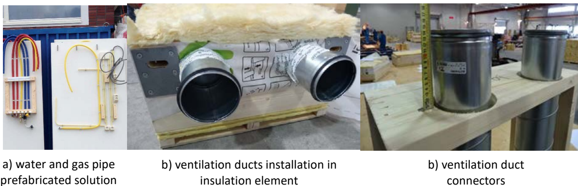
FIGURE 3 MODULAR PIPE INSTALLATION
