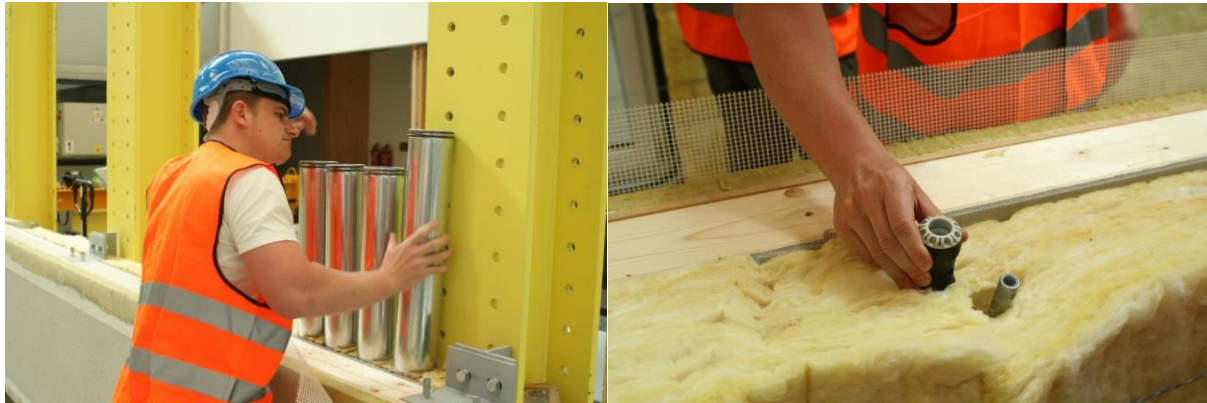
Fig. 1 Preparation for the assembly test in the Czech Republic– fixing the connection elements for the air ducts and the piping.
