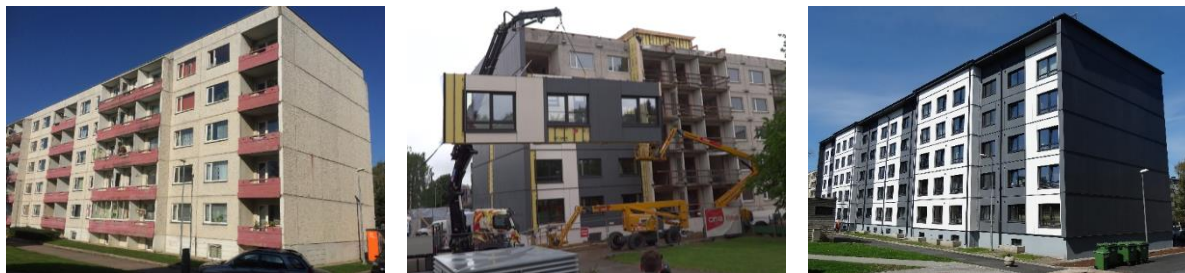
FIGURE 1. PHOTO OF THE PILOT BUILDING BEFORE (LEFT), DURING (MIDDLE) AND AFTER (RIGHT) THE RENOVATION.
