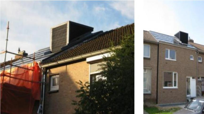
Figure 34: Prefabricated installation platform placed in an integrated PV roof.
