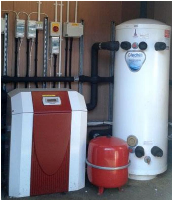
Figure 5: Example of a heat pump and a buffer tank for utility buildings.
