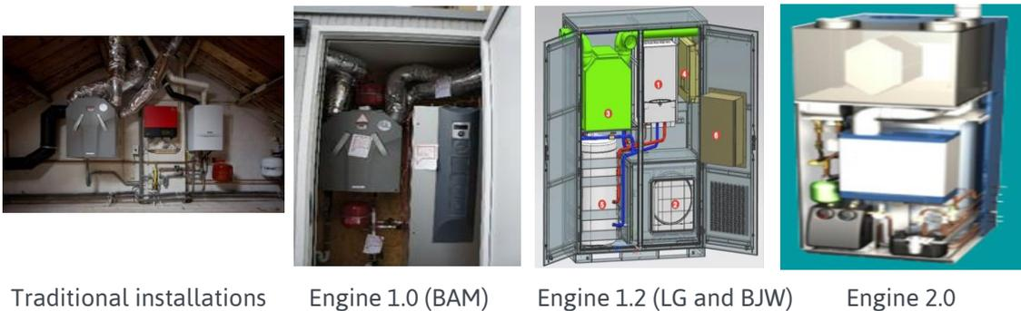
Figure 33: Development of traditional building services into engines (1.0,1.2, 2.0).
