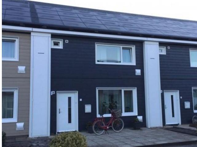
Figure 9: Examples of first generation engines developed in Energiesprong (Volker Wessels), engine in portal next to front door.
