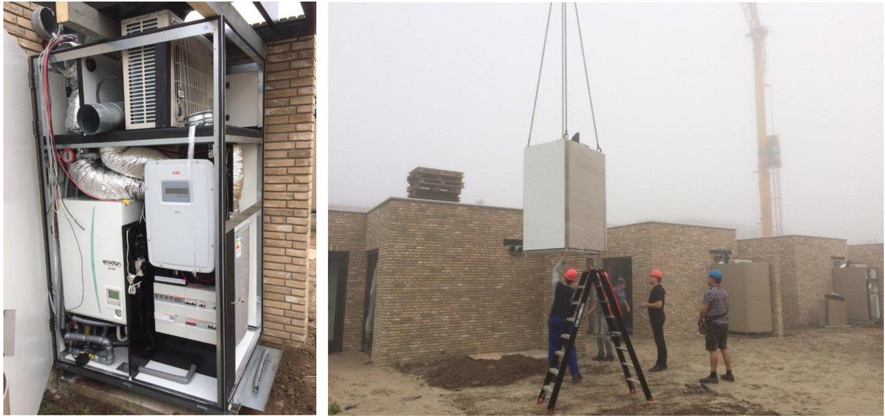
Figure 11: Energy Zero installations module applications in real-life environment (<http://factoryzero.nl/>).
