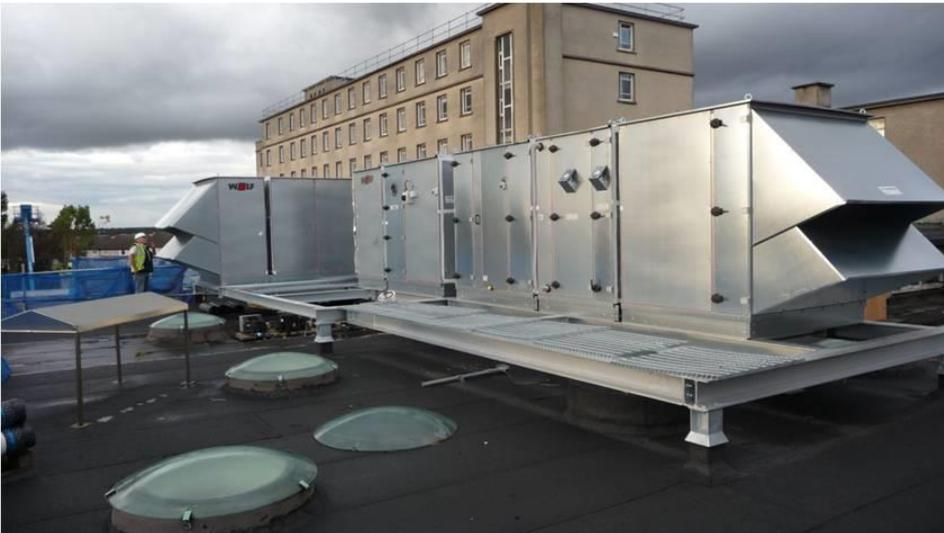
Figure 26: Modules of the AHU units mounted in one steel framework.
