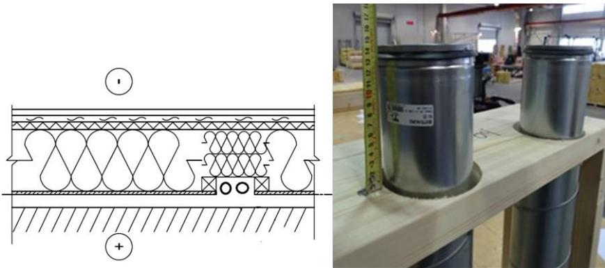
Figure 29: Example of the integrated shaft for HVAC pipes, ducts and distribution channels inside a prefabricated building module (wall panel).
