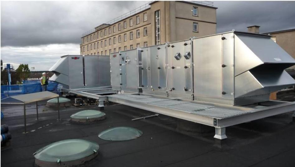
Figure 4: Example of a stand-alone AHU unit for commercial buildings.
