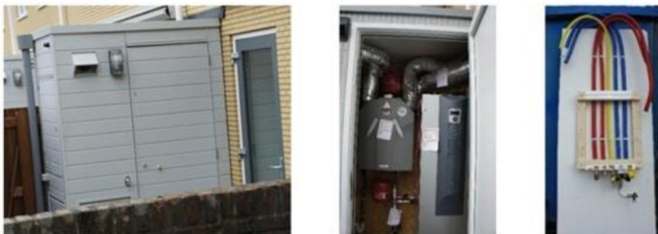
*Figure 8: Examples of first generation engines developed in Energiesprong (BAM), modular HVAC unit (left), modular HVAC unit with heat pump and ventilation heat exchanger (middle), and gas boiler installation (right). No miniaturization yet.*
