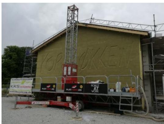
Figure 39: Picture of 3D milled design on facade (Source: Robot At Work)
