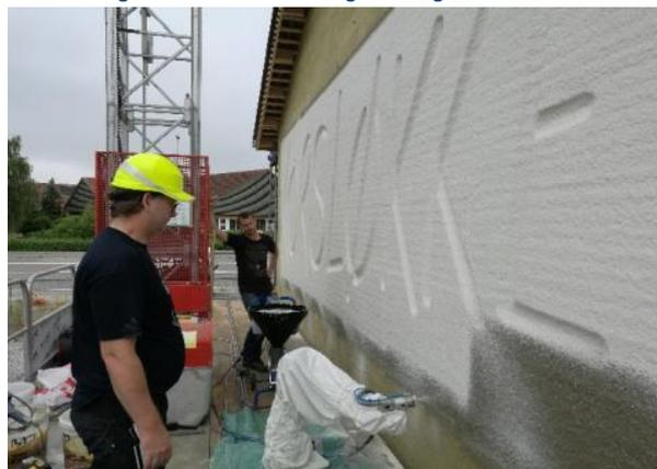
Figure 43: Mortar pump and spray gun
