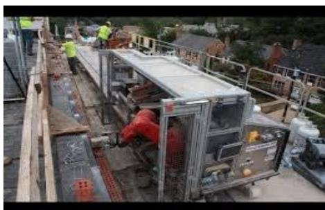
Figure 35: Robot laying bricks (source: Autodesk university)
