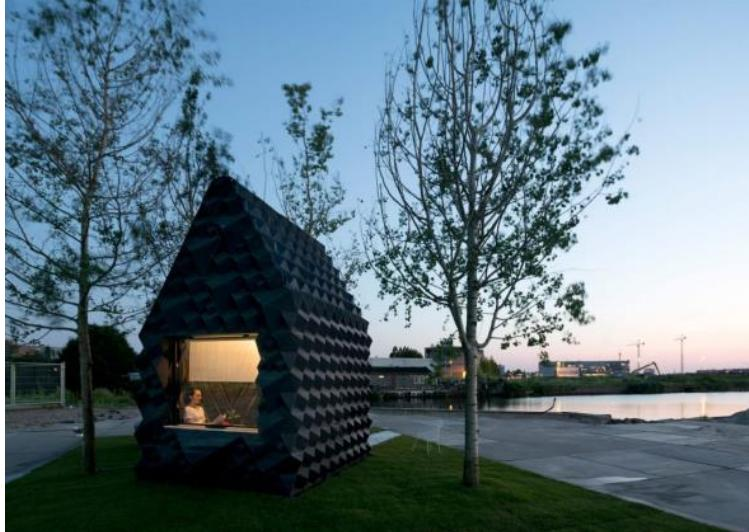
Figure 37: 3D printed cabin Source (DUS Architects)
