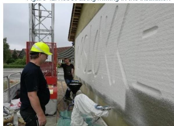
Figure 43: Mortar pump and spray gun
