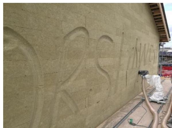
Figure 41: Robot doing milling in the insulation
