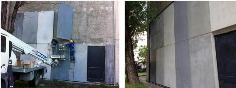
Figure 11: Test façade at Politecnico di Milano: erection of the façade (left) and the completed façade (right) [9].
