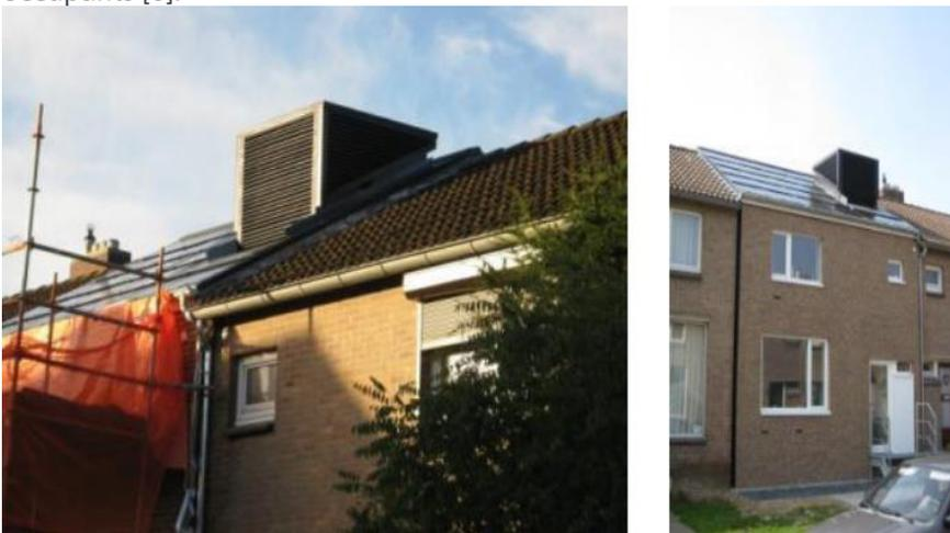
Figure 22: Prefabricated installation platform placed in an integrated PV roof [8].
