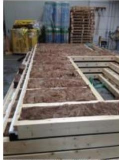
Figure 3-3 Timber-framed construction
