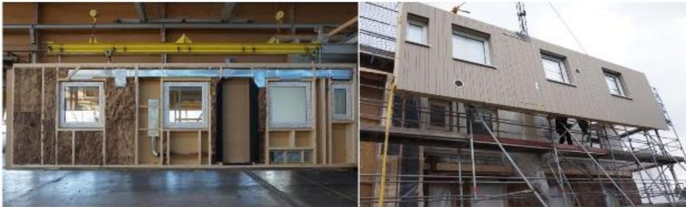
Figure 16: Parts of the ventilation system installed in the wall during prefabrication (left) and installation of the prefabricated wall element on the demo site (right) [15].
