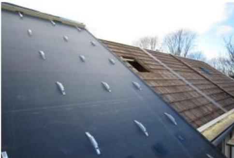
Figure 3-4 Roof with mounting clips for PV panels
