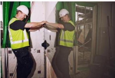
Figure 3-6 Kitchen, mounting glass wall panels
