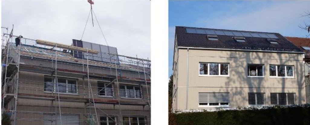
Figure 23: Installation of the solar collector (right) and final view of the surface-integrated solar collector [15].
