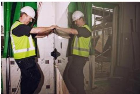
Figure 3-6 Kitchen, mounting glass wall panels
