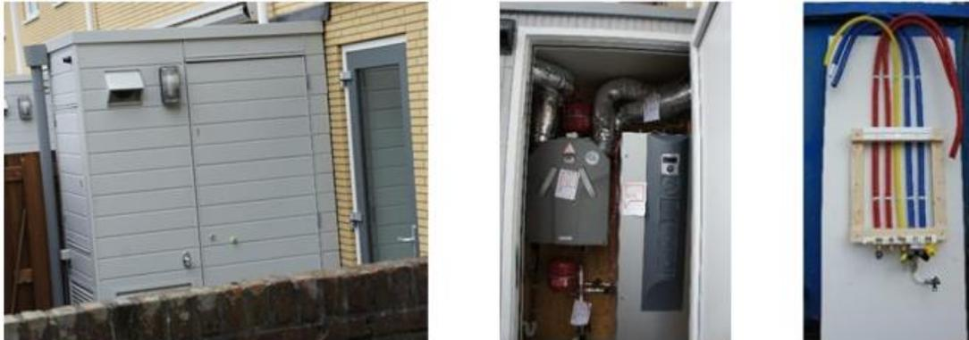
Figure 24: Example of modular HVAC unit (left), modular HVAC unit with heat pump and ventilation heat exchanger (middle), and gas boiler installation (right) [8].
