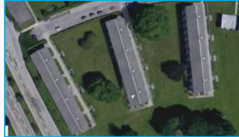
Residential district renovation in Odense, DK
