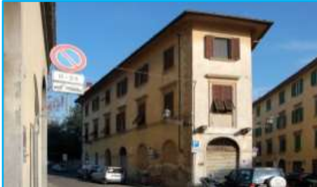
Deep renovation of historic residential building in Florence, IT
