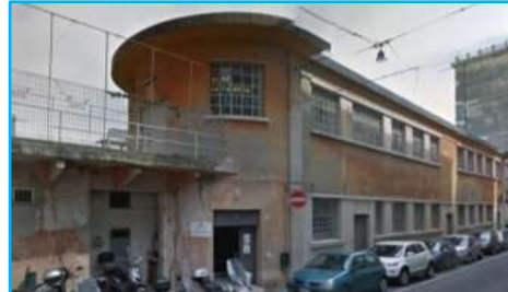
Deep renovation of historical nursery building in Genova, IT
