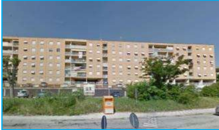
Deep renovation of residential building in Ancona, IT
