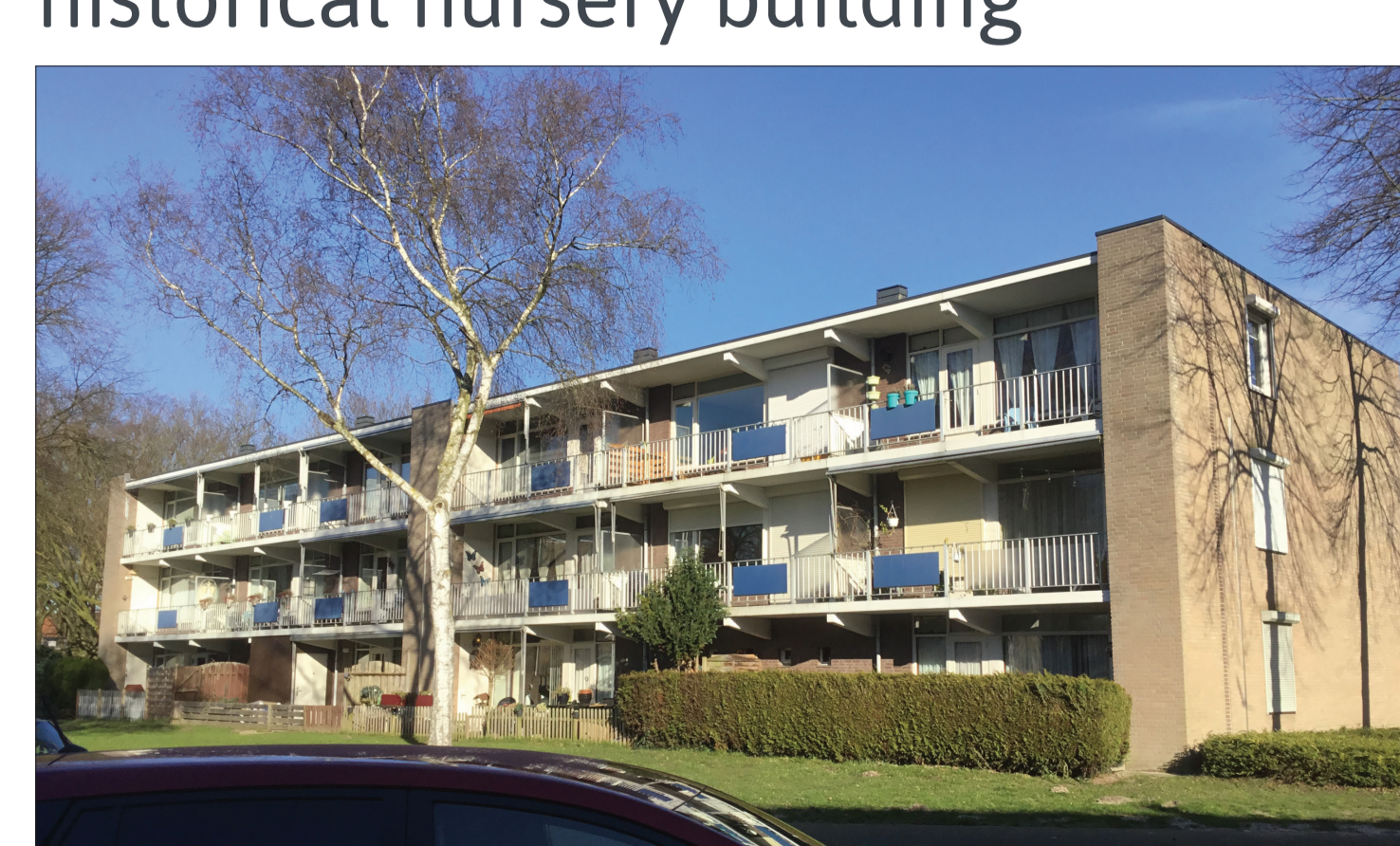
Tilburg NL - Deep renovation of portico flats
