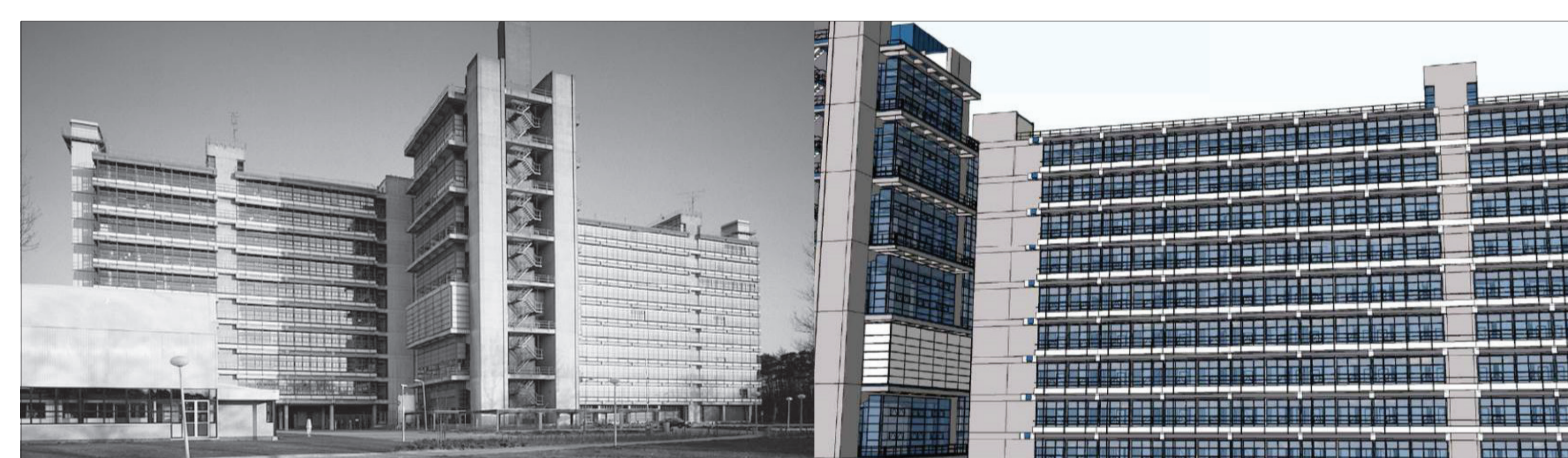
Enschede NL - Transformation of university building to student housing
