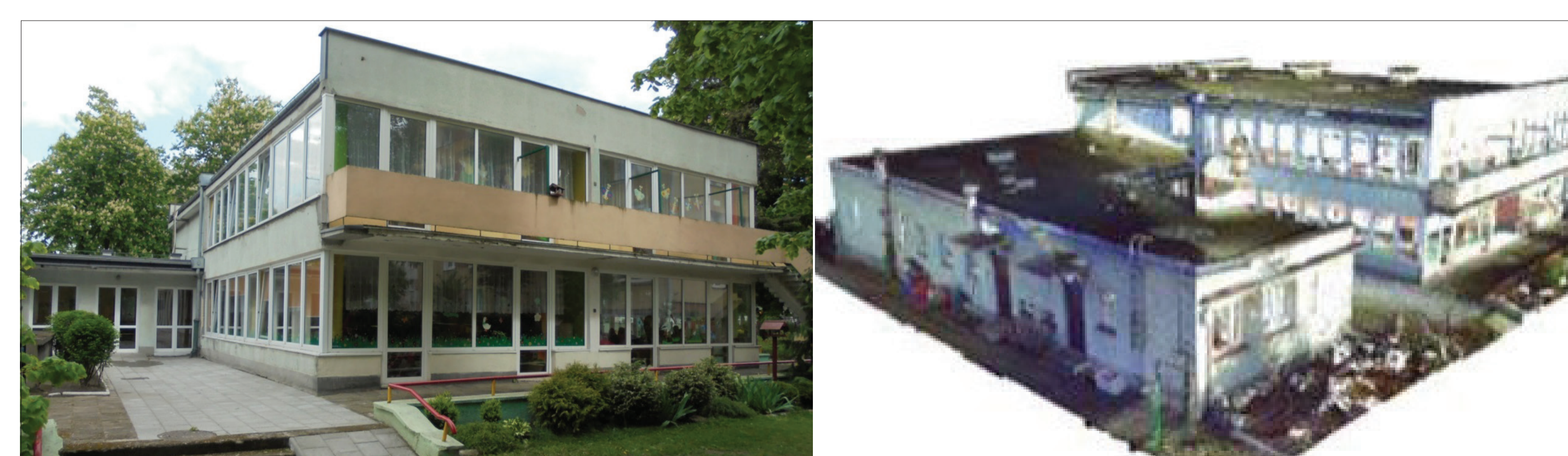
Gdynia PL - Deep renovation of public nursery building
