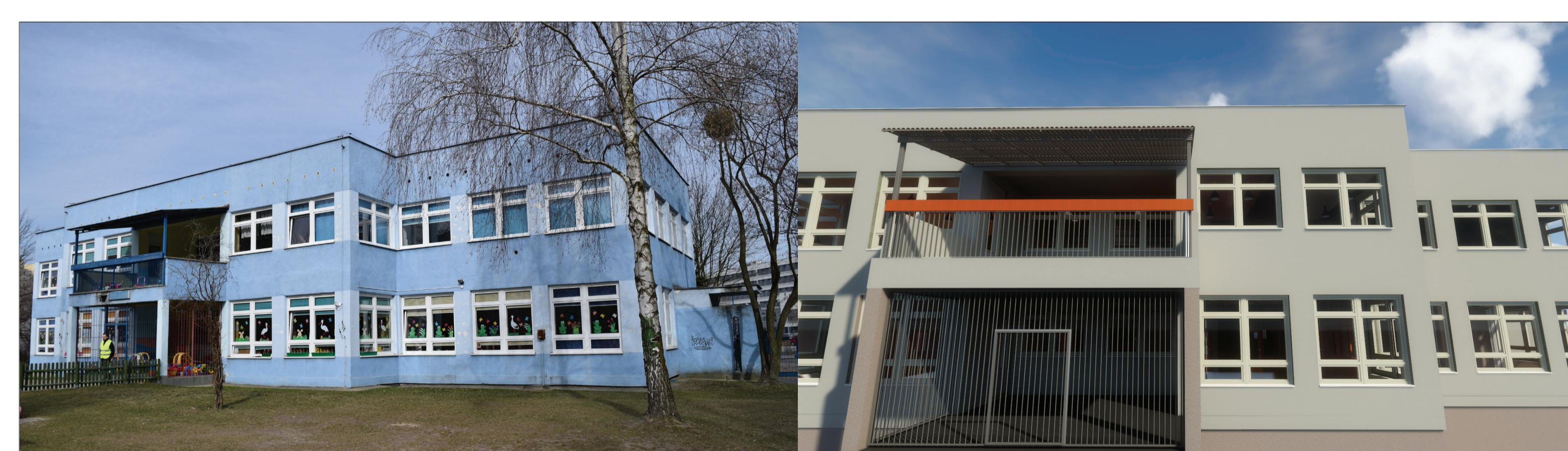
Warsaw PL - Deep renovation of public nursery building
