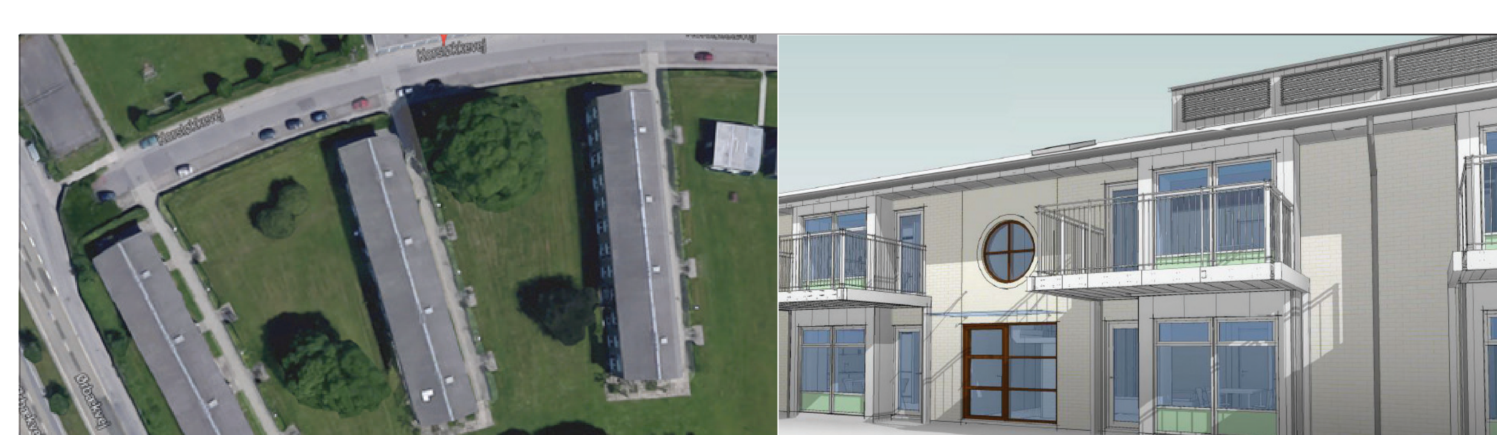
Odense DK - Residential district renovation
