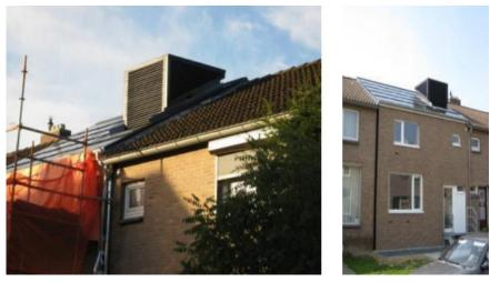
Figure 34: Prefabricated installation platform placed in an integrated PV roof.
