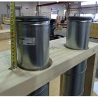
Figure 29: Example of the integrated shaft for HVAC pipes, ducts and distribution channels inside a prefabricated building module (wall panel).
