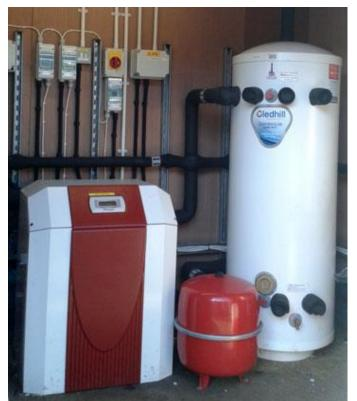
Figure 5: Example of a heat pump and a buffer tank for utility buildings.
