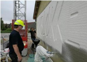
Figure 43: Mortar pump and spray gun
