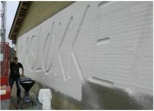
Figure 42: Robot is rendering with mortar
