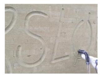
Figure 40: Robot doing design milling
