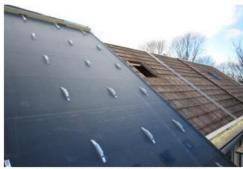
Figure 3-4 Roof with mounting clips for PV panels
