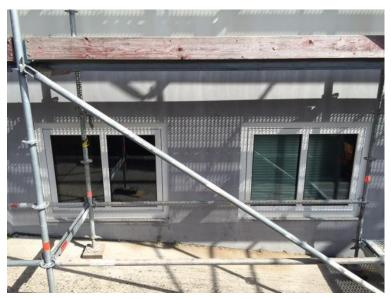
Figure 19: A2PBEER Smart window prototype installed on a demonstration site in Malmo, Sweden.
