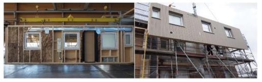
Figure 16: Parts of the ventilation system installed in the wall during prefabrication (left) and installation of the prefabricated wall element on the demo site (right) [15].
