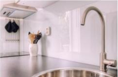
Figure 3-7 Result, glass wall panels
