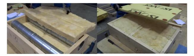
Figure 5: First prototypes of MORE-CONNECT prefabricated panels [8].
